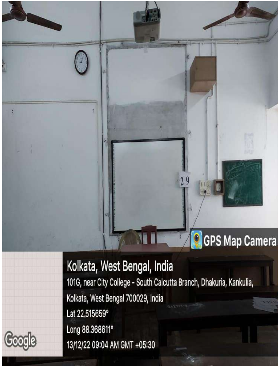
Room No. 29 - Projector, Smart Board and Wi-Fi
