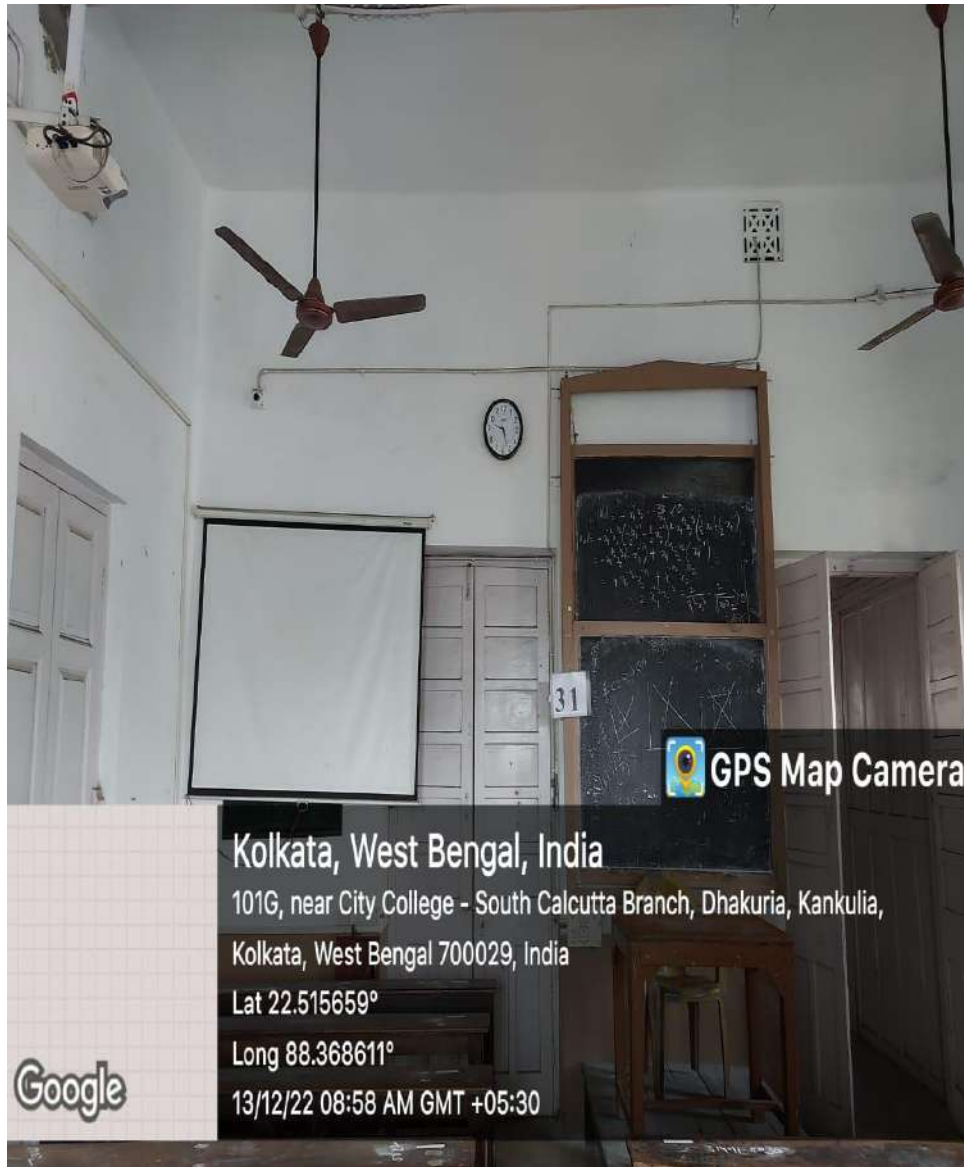
Room No. 31 - Projector and Wi-Fi
