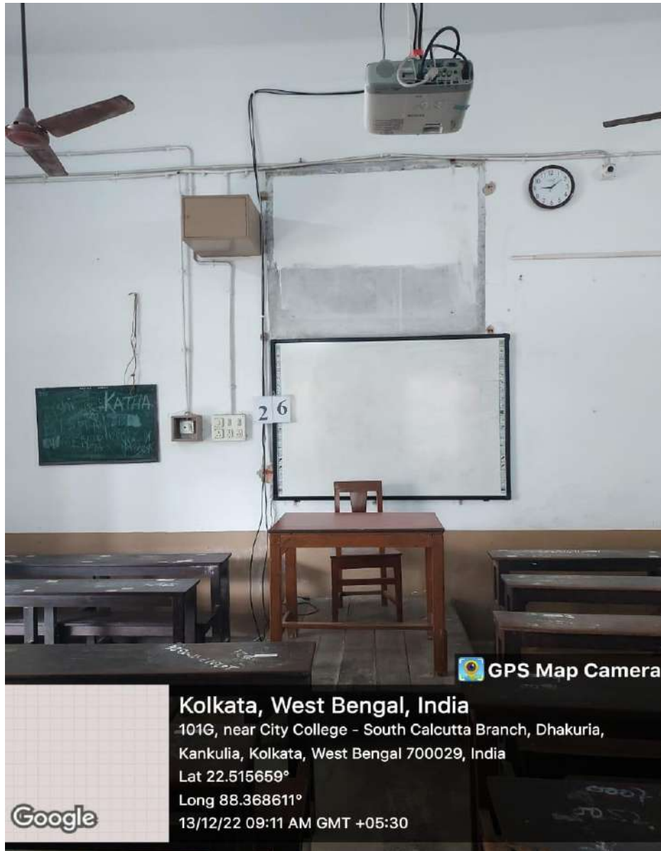
Room No. 26 - Projector, Smart Board and Wi-Fi
